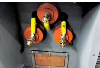
Conduit box with standoff insulators
